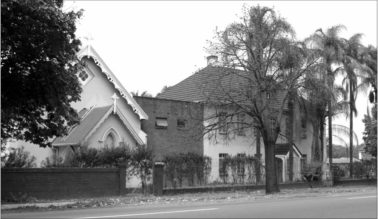
ABOVE 1875 Loop Street, Pietermaritzburg. On the left is the former St Mary's Church, St Mary's Chapel in 2002. On the right is Bishop Allard's house, the probable first home of Bishop Charles Jolivet and, therefore, first home of St Charles' Catholic Grammar School for Boys, established on 26 July 1875. (This photograph dates 2001.)
